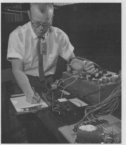
to meet stringent design specifications after periods of storage. Special test equipment like this QT-115 is designed by QA when no commercial equipment will make the necessary measurements.
